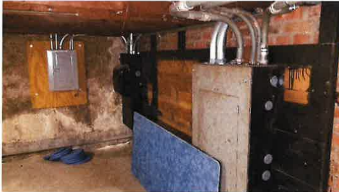
Remnants of original electrical service opposite wall of current
